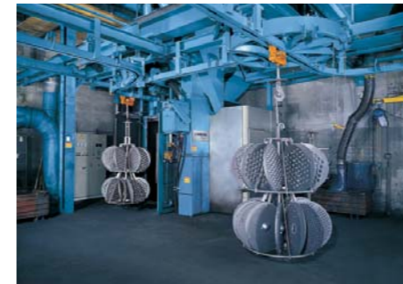
Customised monorail system with switch points
